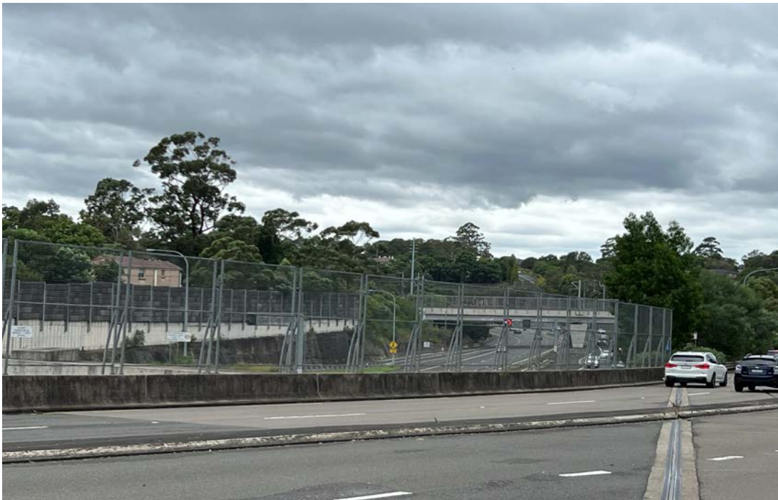
Figure 8: View east along motorway cutting from Beecroft Road overbridge, showing depth of cutting. In left foreground are the tops of the concrete pillars on which it is proposed to erect the signage.
